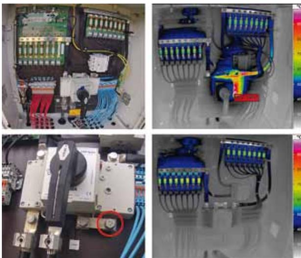
A string connection box (SCB) with a loose screw connection. Even if the position of the defect is known, it cannot be detected visually. Thermogram on the top right: a loose screw is causing a temperature rise of 150 K. This means acute danger of fire. The box needs to be taken out of operation and repaired immediately. Image bottom right: temperature distribution of a fault-free SCB.
